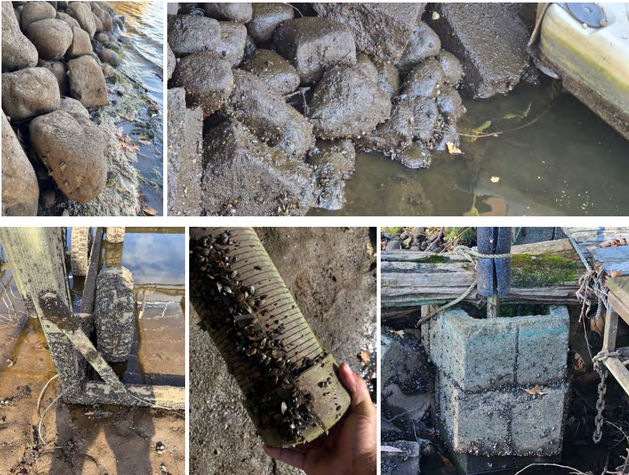
Five of the numerous photos taken by OLID members during the October 1, 2025 Dam Inspection drawdown.
